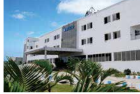
Rudrapur Plant (Green Building)
