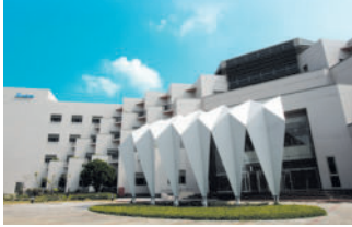
Tainan Plant (Diamond-rated Green Building)
